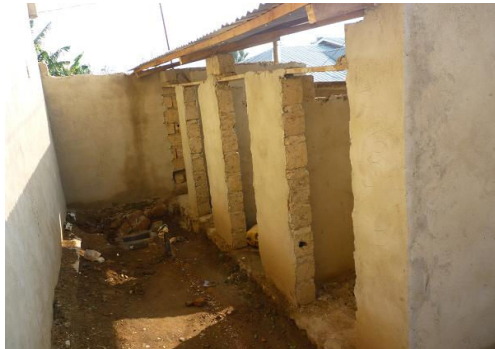
Work on toilet block.
